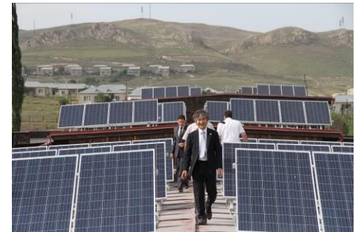
Installed solar panels on the roof of school
