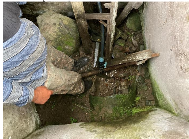
Inside of the valve manhole
