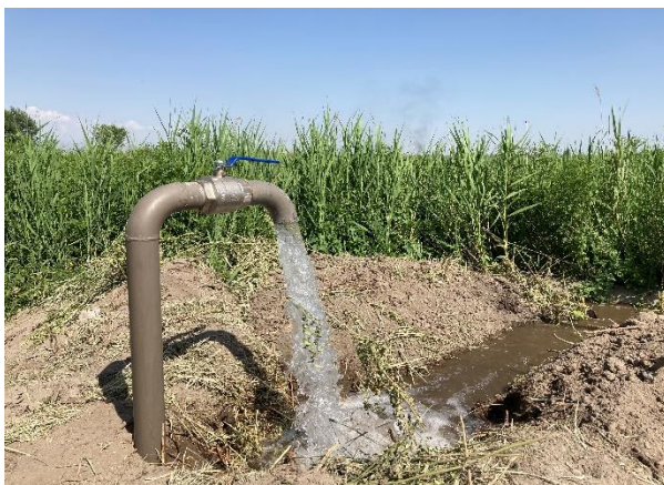
The newly installed irrigation system
