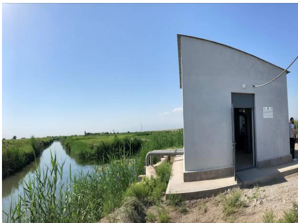
The newly established pump station
