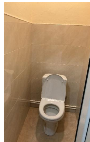
Newly installed toilet
