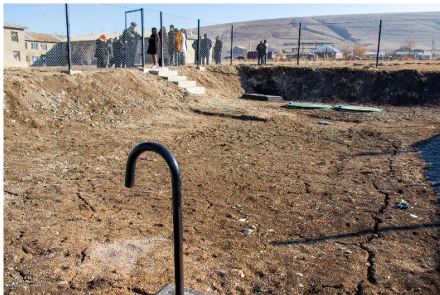
Newly constructed sewage system
