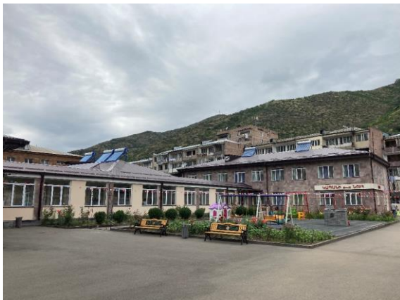
The renovated building
