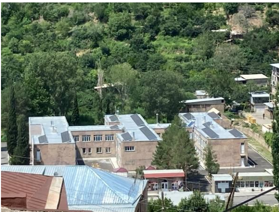
Installed solar panels on the roof of building
