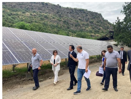
Demonstration of the photovoltaic station
