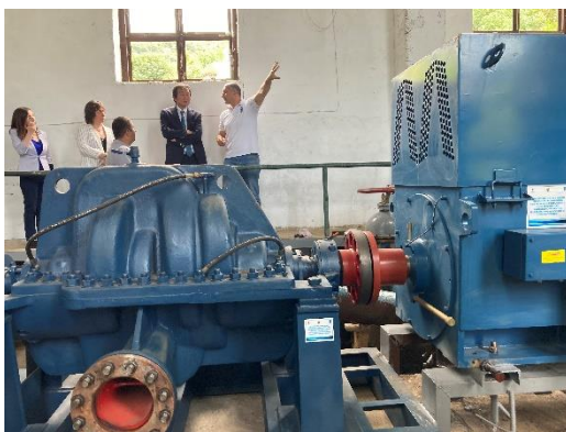
Presentation of the pump station
