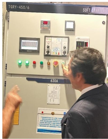
Ambassador AOKI switching on the pump
