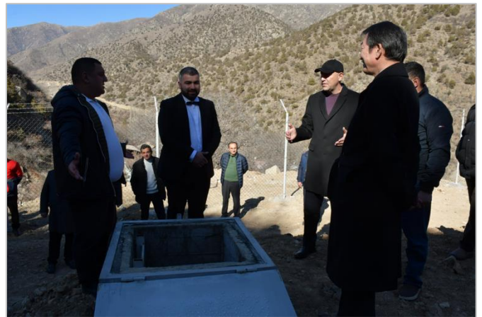
Ambassador Aoki inspecting the newly installed water pipe
