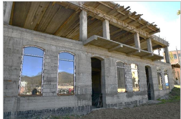
Windows and roof installed through this project
