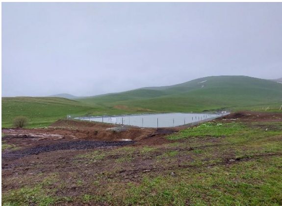
Chambarak Water Reservoir
