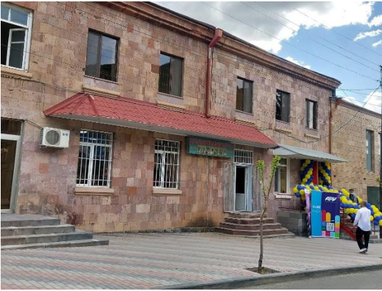
Renovated youth center
